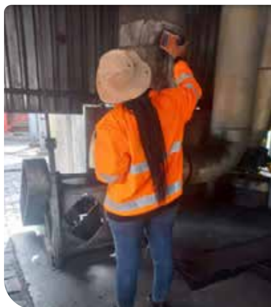
Coal boiler stack air emissions sampling
