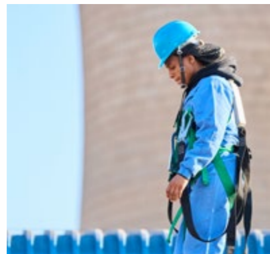
Ratchel Vatakati (Electrician), inspecting the Colcom Solar Project
