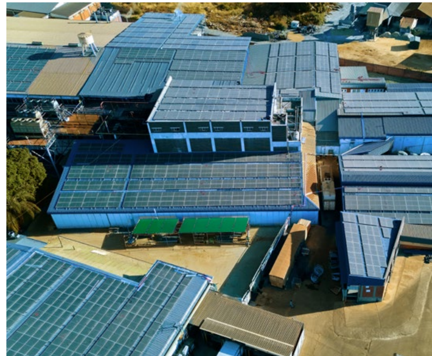
Colcom Complex Coventry Road - Solar Installation
