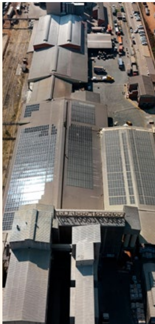
National Foods Aspidale - Solar Installation
