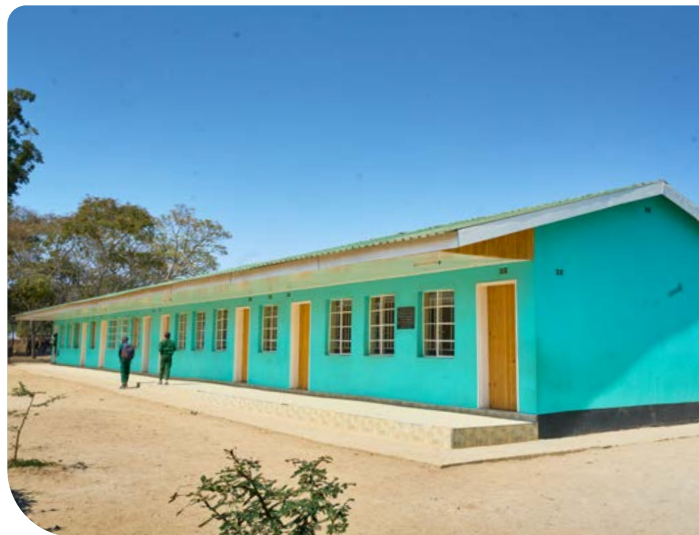
St Marnock’s School Block
